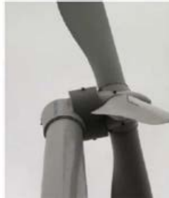
gearless generator with magnets of rare earths
