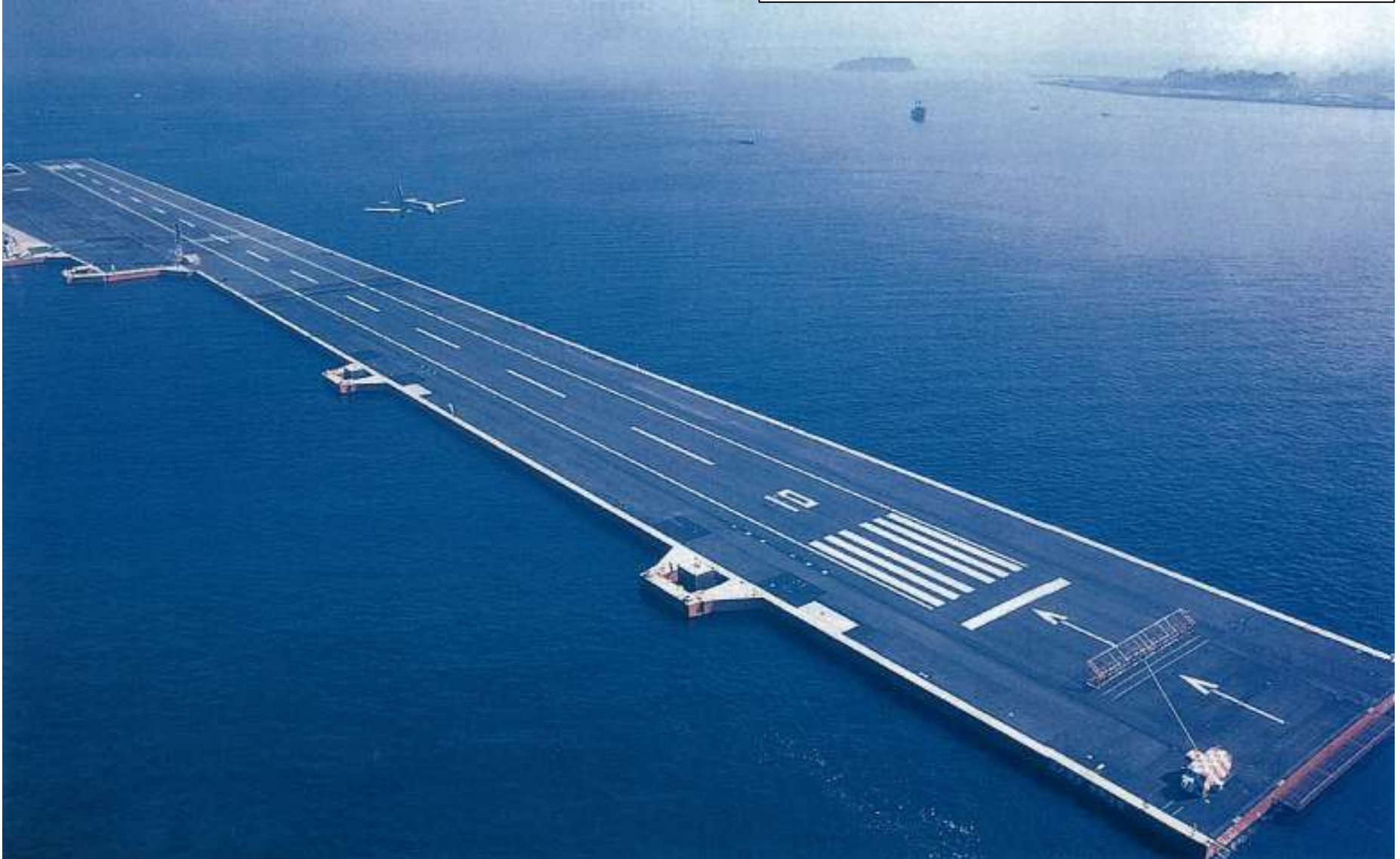
Test Model of Mega Float, constructed in cooperation with Japanese Shipping Companies
